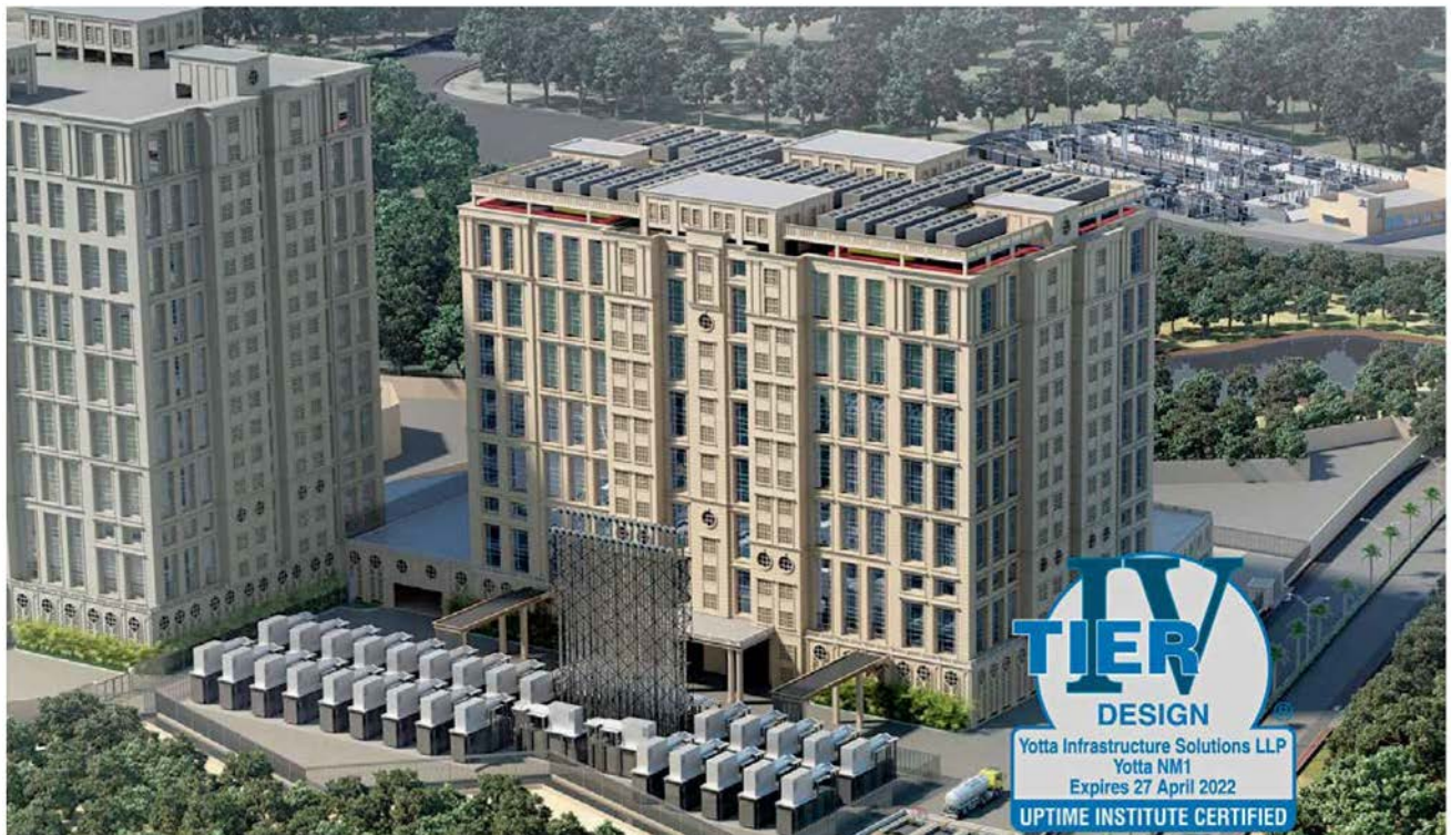
Yotta NM1 – World’s Second-Largest & Asia’s Largest Uptime Institute Tier IV Design Certified Data Center 8,20,000 sq. ft area | 7200 Racks | 50 MW Power | 1.4 Power Usage Efficiency (PUE)
